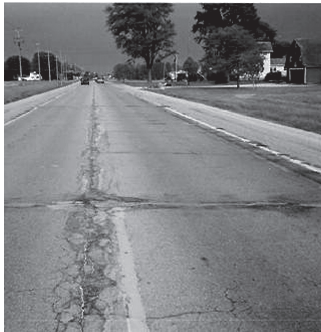
Figure 2.3 Reflection cracking in HMA overlay of PCC pavement (courtesy Antigo Construction, Inc.)
